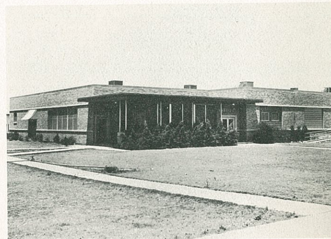
EAST PRIMARY CAFETERIA
